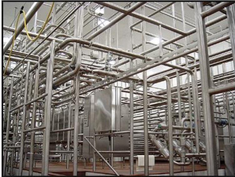
Fig. 5. Pipework Which Needs to be Mapped Before it can be Dismantled
