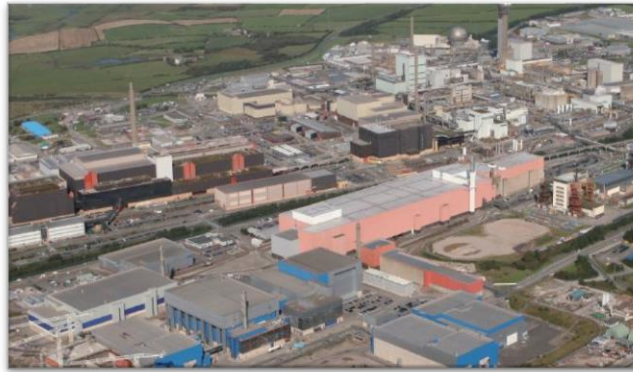
Fig. 1. The Sellafield Site in Cumbria, UK
